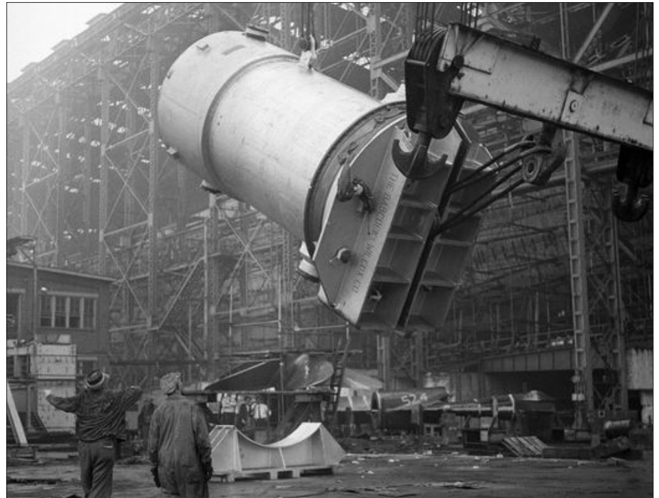
A crane hoists a part for a nuclear reactor in 1959 at the New York Shipbuilding yard in Camden. The city was once brimming with manufacturing jobs. (Photo: Associated Press)
